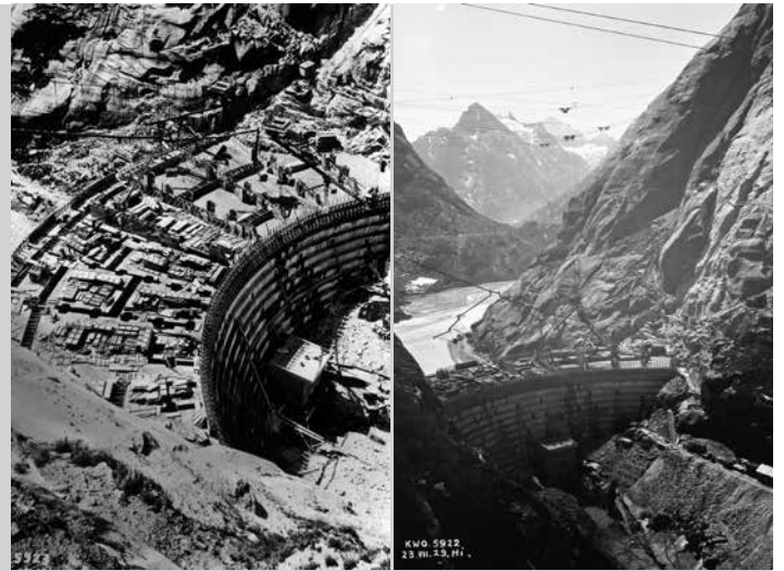
Old Spitallamm construction site
